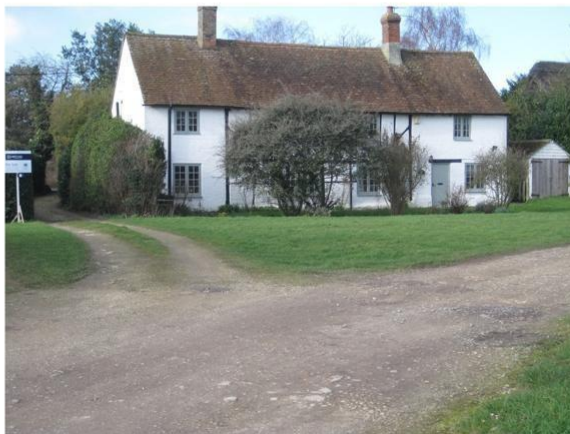
Timber-framed brick & render & tiled house
