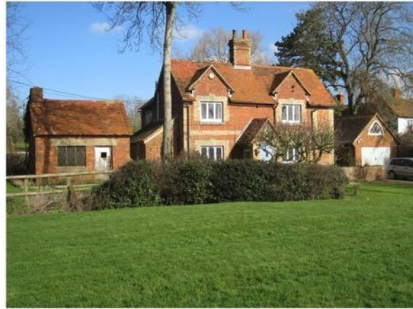
Victorian decorative brick & tile cottage
