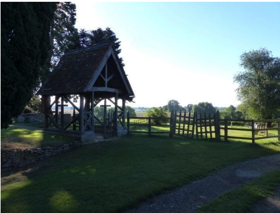
Lych gate at St Lawrence's Church, Toot Baldon; views towards the Chilterns beyond
