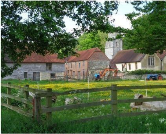
Baldon House barns, stables with St Peter's beyond
