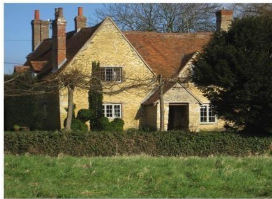
North side of the Green: No 19 The Green
