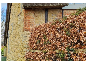
Figure 43: Limestone rubble with some timber framing and brick infill.
