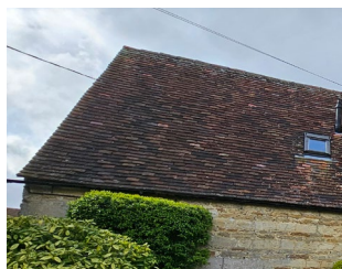
Figure 52: Hand made clay plain tile roof.
