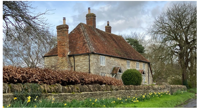
Figure 23: Limestone building with clay tiled hipped roof and brick chimney stacks with clay pots.
