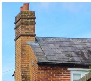
Figure 56: Slate tile roof.
