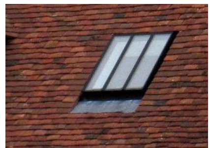
Figure 67: Conservation metal rooflight laid in with the tiling.
