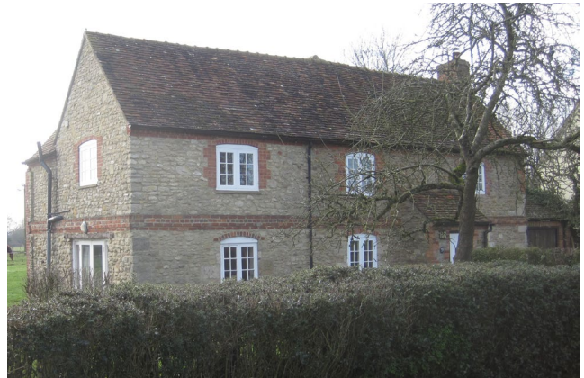
Figure 90: Rubble stone cottage with brick dressings, located on the eastern end of southern Green, Marsh Baldon.
