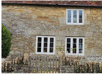
Figure 60: Vertical panelled white painted casement windows.
