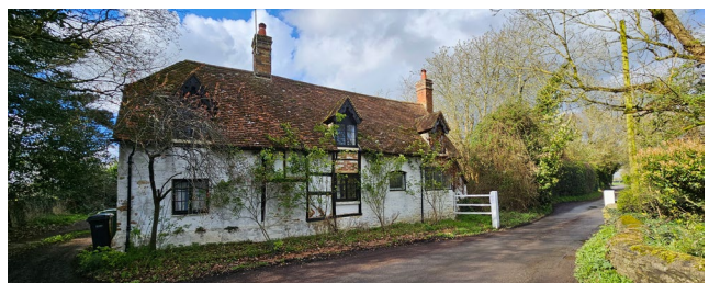
Figure 26: Combination of colourwashed limestone rubble, timber framing and painted brick with red brick detailing between the central dormer. The roof is half-hipped with clay tiles, small pitched dormers and brick chimney stacks with clay pots.
