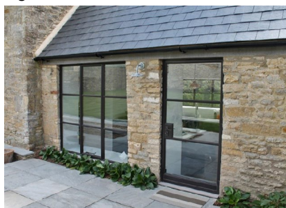
Figure 69: Modern metal window.
