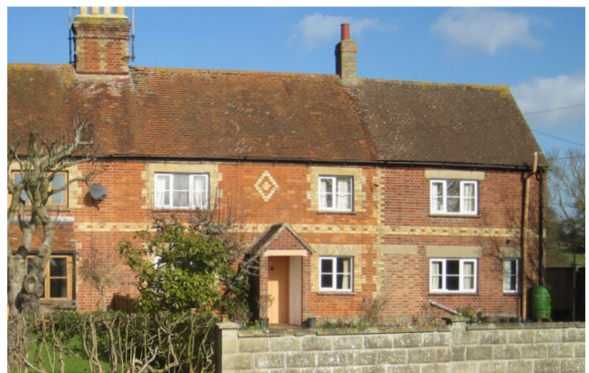
Figure 24: Terraced, red brick cottages with yellow brick detailing, a clay tiled pitched roof and a pitched roof porch.
