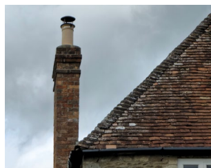
Figure 53: Clay plain tile roof details.
