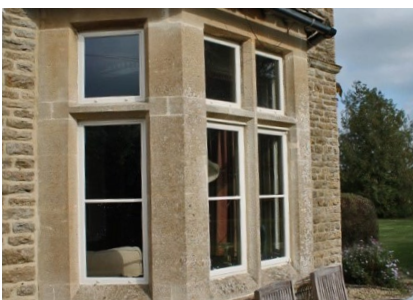
Figure 65: Metal windows in stone surrounds - a traditional way to fenestrate with dressed stone features
