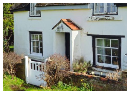
Figure 82: Pitched roof porch example.
