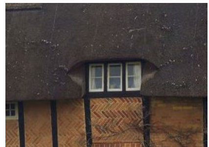
Figure 64: Small timber framed vertical windows in an eyebrow dormer.
