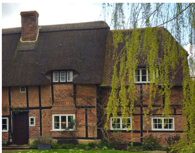
Figure 32: Local example of a side extension to a thatch property, Marsh Baldon. The extension sits behind the property line and matches the materials and design of the existing building.
