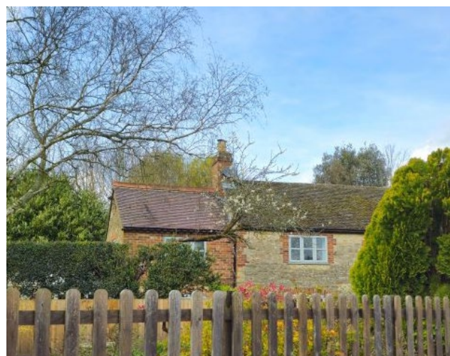
Figure 33: Local example of a side extension to a stone property. The extension is subordinate to the main building, whilst not using the same materials the brick colour matches that of the dressings on the main house which helps to maintain visual harmony.
