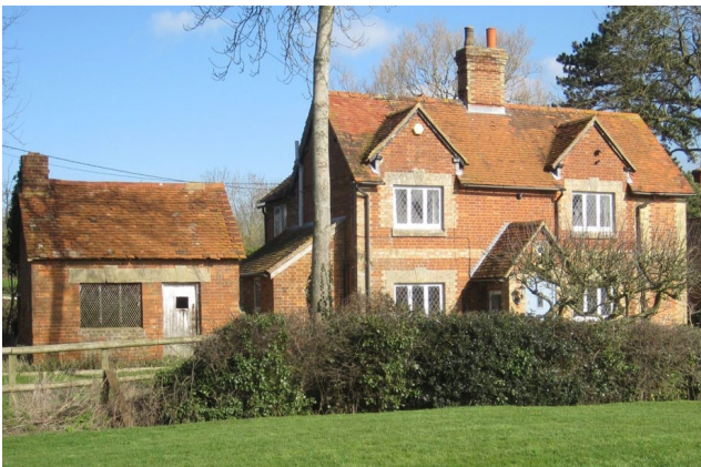
Figure 85: Brick cottage with brick dressings located on the north side of The Green, Marsh Baldon.
