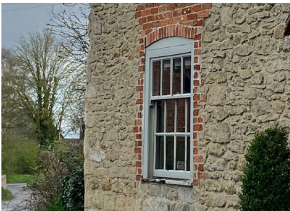
Figure 62: Painted timber panelled sash window with brick dressing.
