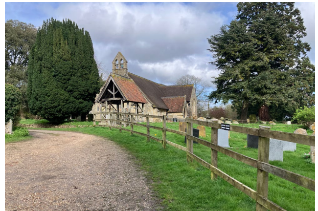
Figure 22: Grade II* listed St Lawrence Church.
