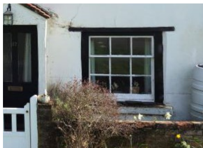
Figure 63: Painted timber panelled sash window with dark timber frame.
