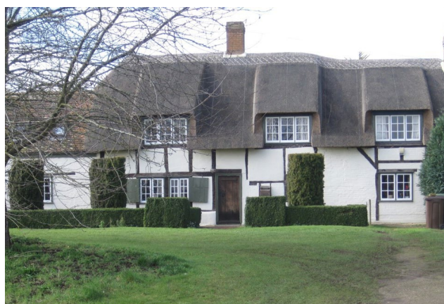
Figure 84: Timber-framed house with rendered panels, a thatched roof and extended at either end. Located on the south west corner of The Green, Marsh Baldon.
