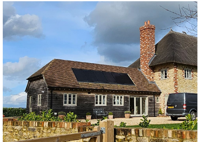
Figure 111: PV panels on the roof of a side extension to a property in the Baldons.
