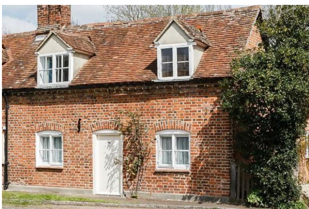
Figure 83: Nuneham Courtenay cottages, in red brick with clay tile, pitched roof and small, pitched roof dormers.
