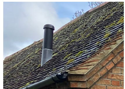
Figure 76: Metal stove pipe.
