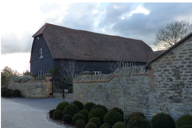
Figure 95: Barn conversion in Toot Baldon.
