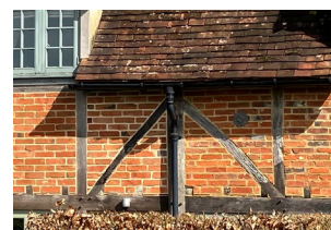
Figure 42: Timber frame with brick infill.
