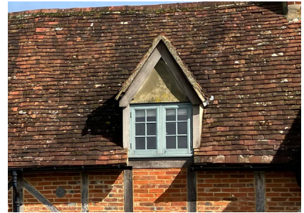
Figure 61: Painted timber panelled casement window in a pitched dormer.
