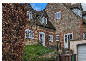
Figure 45: Limestone rubble with red brick dressings.
