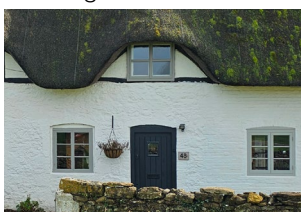
Figure 47: Colourwashed limestone rubble with painted brick extension to the right.
