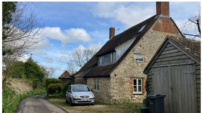
Figure 25: Limestone house with small amounts of red brick detailing and a steeply pitched roof with lidded dormer window and brick chimney stacks.
