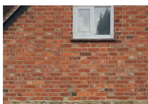
Figure 44: Flemish bond red brick in varying shades
